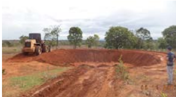
Figure 5 - Containment basin in Curvelo
